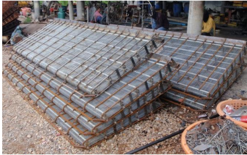
Figure 24 Iron dredge, entrance size 320 cm.
