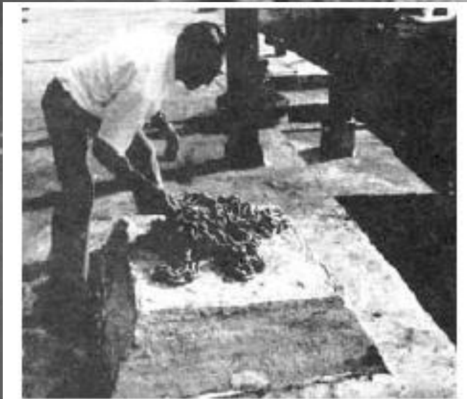
Figure 3: Shaped (545 kg) concrete clump anchor (Western Samoa)
