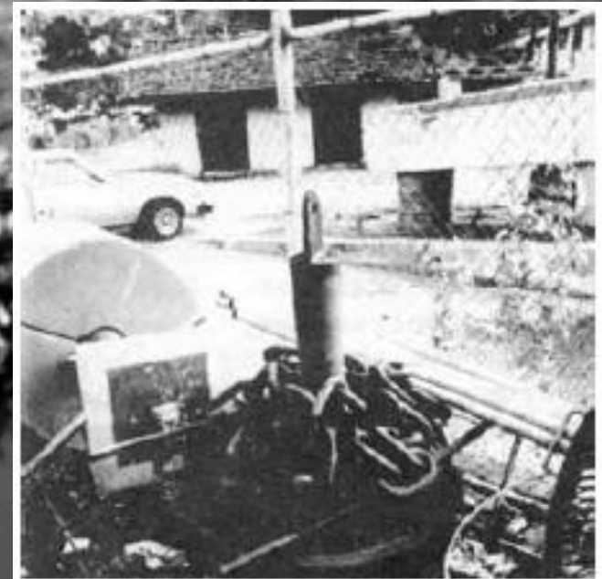
Figure 5: Surplus steel anchor – railway wheel (American Samoa)
